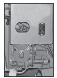
Figure 71: Control valve location.
