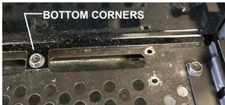
**STEP FOUR:** Install remaining Liner in Center Position in firebox. Attach with 2 DT Screws on top and 2 at bottom.
